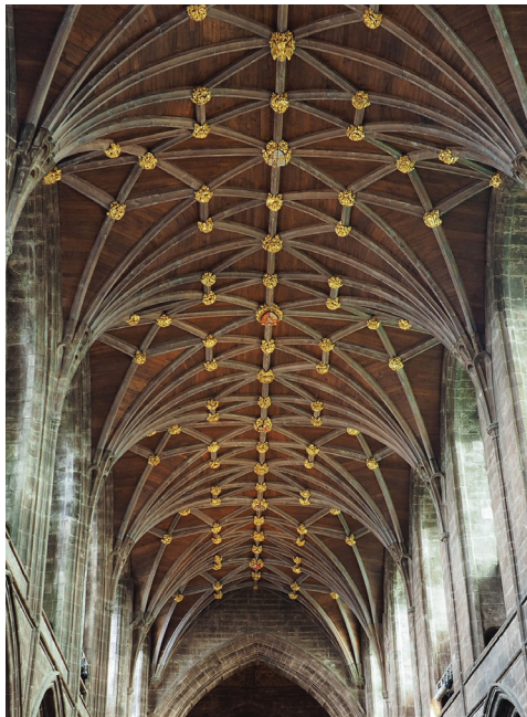
Fig. 6 Tierceron vault, Chester Cathedral, Chester, UK
